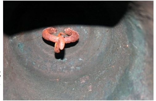
Fig. 5 Looking up inside a bell, showing an example of a cast-in crown staple.
