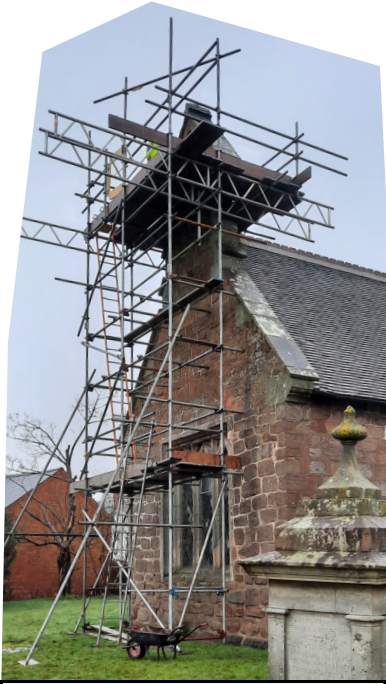
St Peter's west end covered in a web of scaffolding
